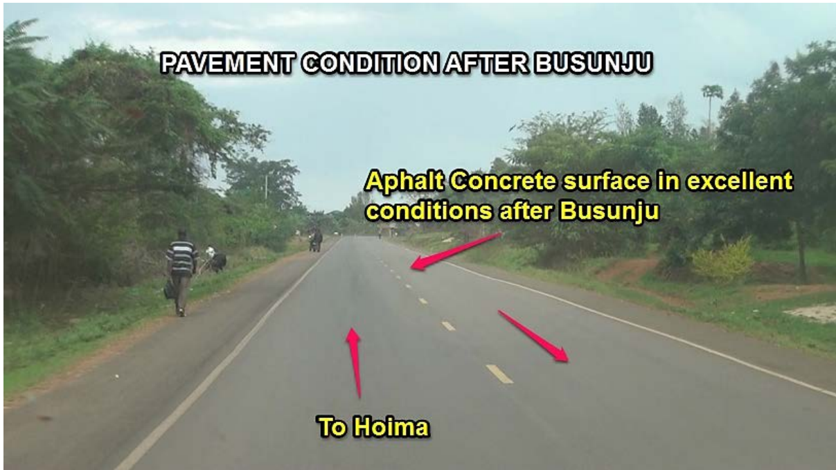
Figure 3: Typical Pavement Condition of Busunju-Hoima Road Section
